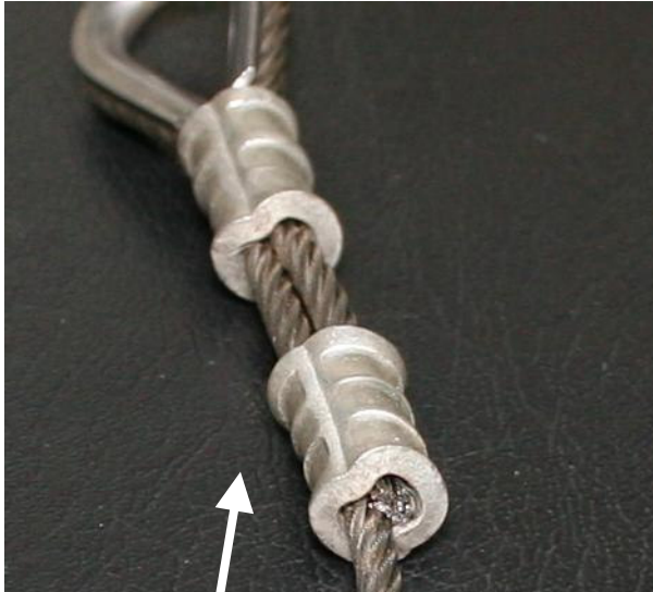
Figure 3 – Inspecting wire and swages for corrosion with heat shrink off.
