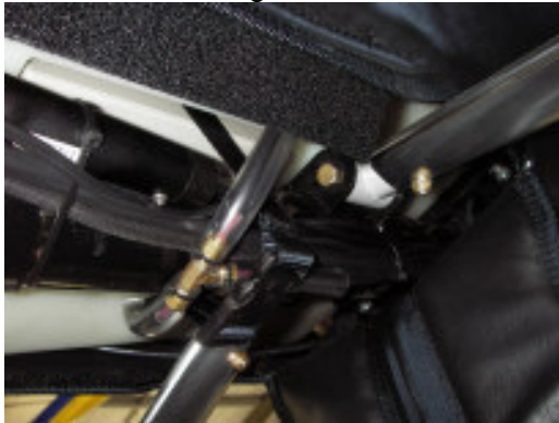
Figure 46 Inspect All Junctions for Oil Leakage
