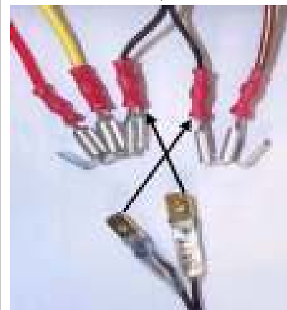
SKYDAT POWER LEADS SHOWN BEFORE CUTTING (LEFT) AND AFTER FITTING (RIGHT) - MARK POSITIVE AND NEGATIVE. (SEE PHOTO)
