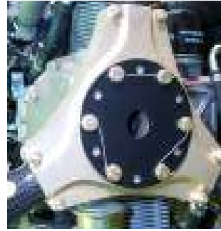
PHOTOGRAPH SHOWS TIE WIRE CORRECTLY INSTALLED
