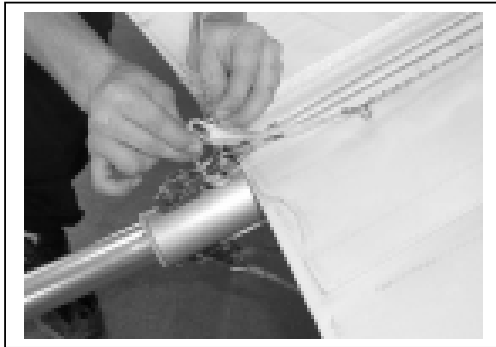
Figure 28 Insert batten
