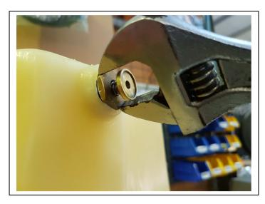
Use adjustable wrench or similar, to remove the draincock assembly.
