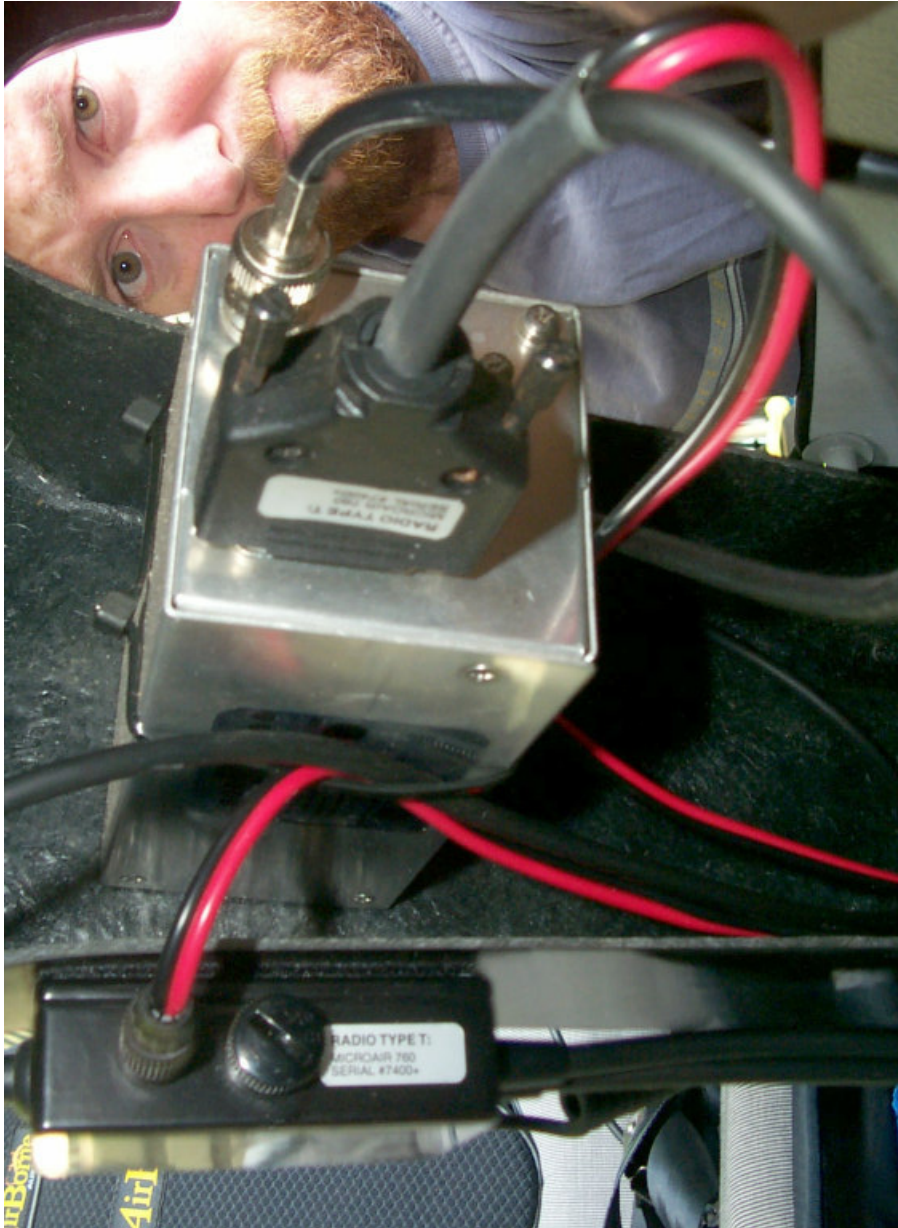
PHOTO SHOWS WIRE ROUTING AFTER INSTALL.
