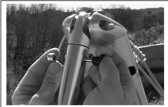
Figure 55 Section 4. Disconnect Base Bar
