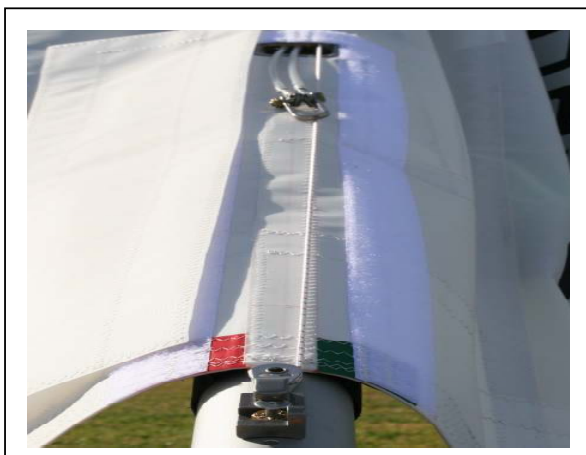
Figure 69 Section 4. De-tension Pull Back Cable
